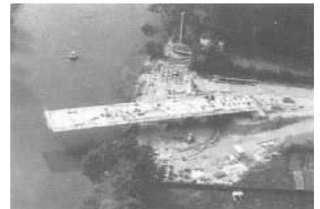
Figure 46: One bridge half nearly completely rotated
