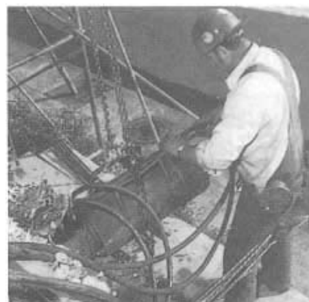
Figure 66: Stressing added tendons
