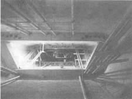
Figure 50: Tendons inside the box
