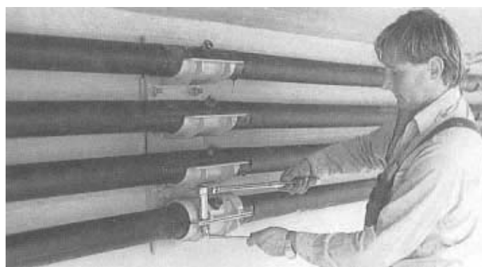
Figure 30: Intermediate tendon supports
