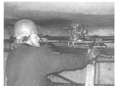
Figure 58: Pushing through strands
