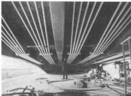
Figure 2: Bridge at Aue; external prestressed bars of the drop-in span
