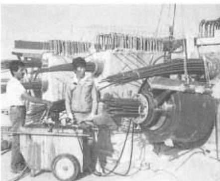
Figure 33: Stressing a VSL tendon
