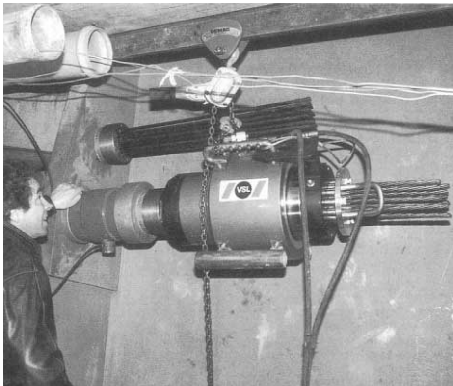
Figure 34 : Stressing of an external tendon equipped with a VSL Load Cell
