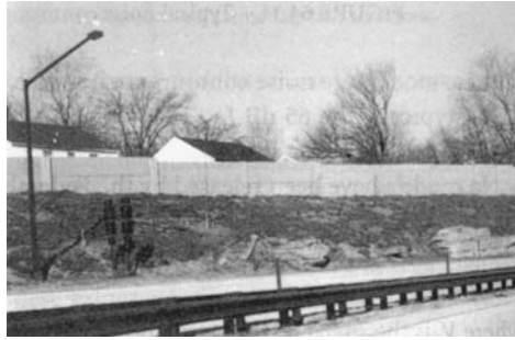
FIGURE 67.12 Typical noise barrier for highway.
