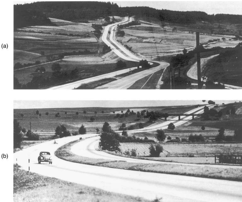
FIGURE 63.16 Example of highways with (a) a long tangent that slashes through the terrain and (b) the more desirable flowing alignment that conforms to the natural contours. (From Transportation Association of Canada, Geometric Design Guide for Canadian Roads , Ottawa, Ontario, 1999. With permission of the Transportation Association of Canada, www.tac-atc.ca .)
