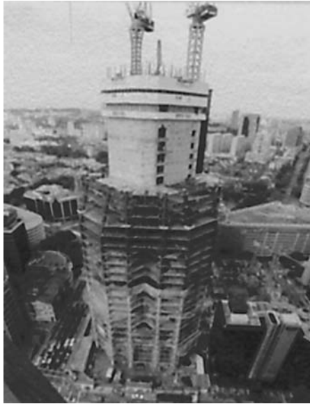
FIGURE 51.6 Composite construction, Republic Plaza, Singapore.
