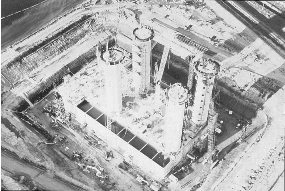
FIGURE 42.2 Wandoo platform under construction in western Australia.
