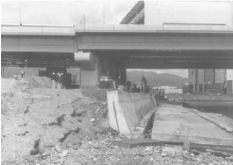
FIGURE 30.7 Liquefaction-caused bridge damage during Kobe earthquake.
