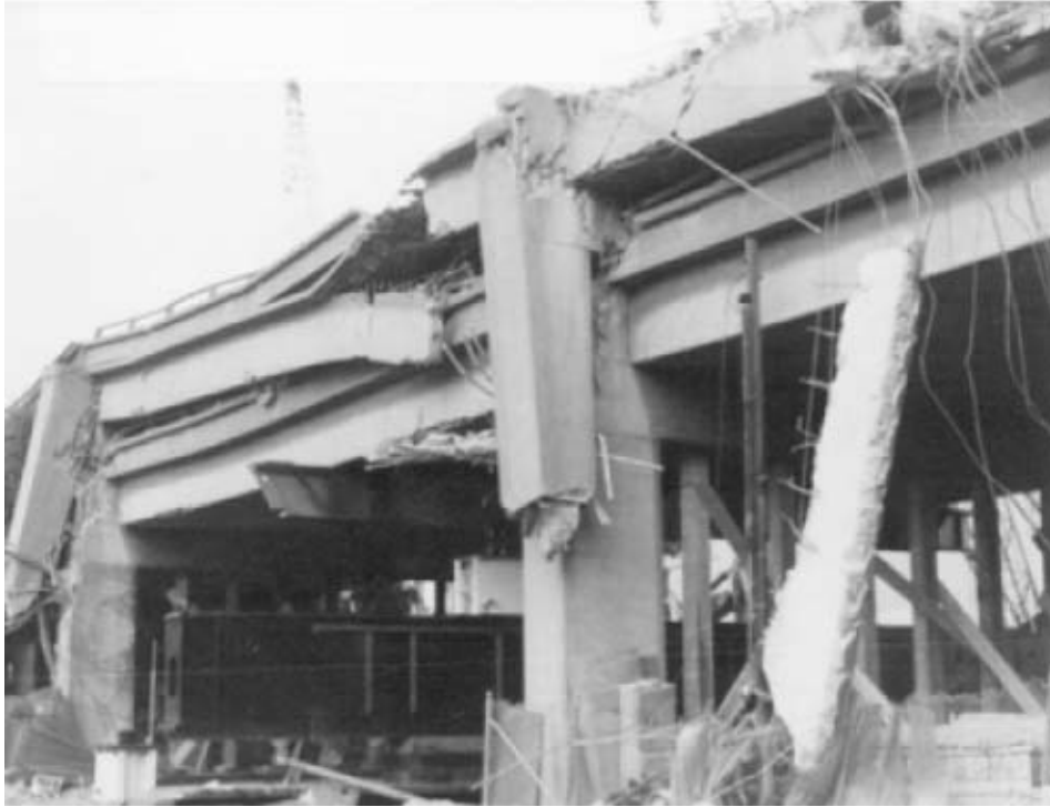
FIGURE 30.28 Damage to Cypress Street viaduct.
