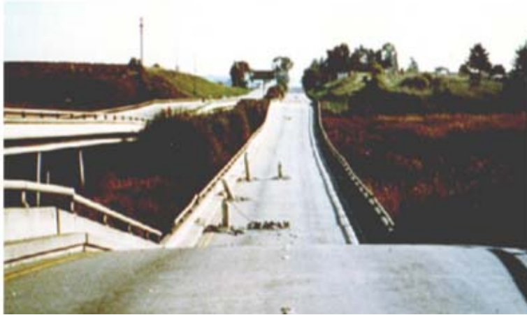
FIGURE 30.26 Piles penetrating the bridge deck.
