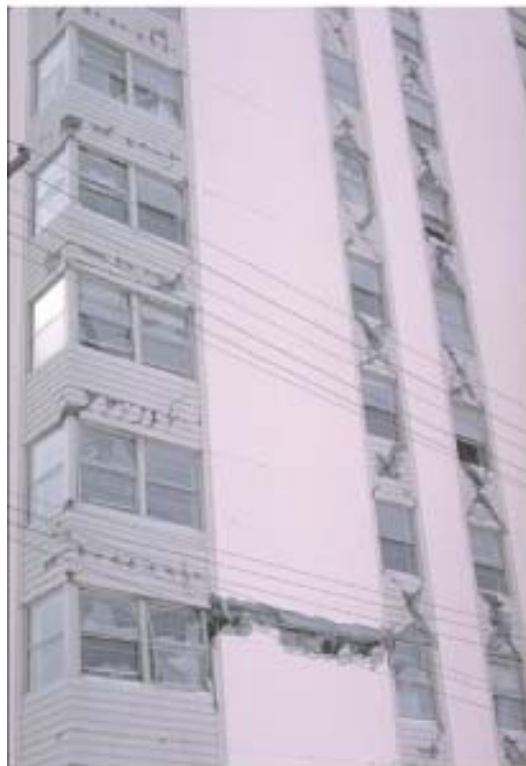
FIGURE 30.49 Damage to north side of Mt. McKinley Apartments. (Photograph by Karl Steinbrugge and courtesy of the Steinbrugge Collection, Earthquake Engineering Research Center, University of California, Berkeley.)
