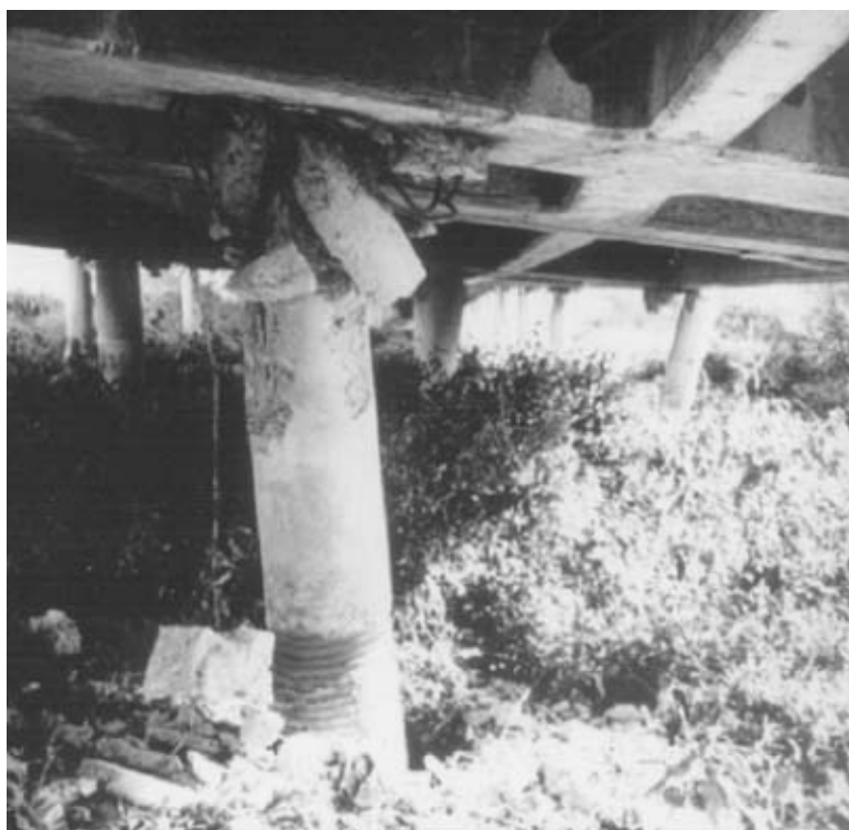
FIGURE 30.25 Broken piles under the bridge.
