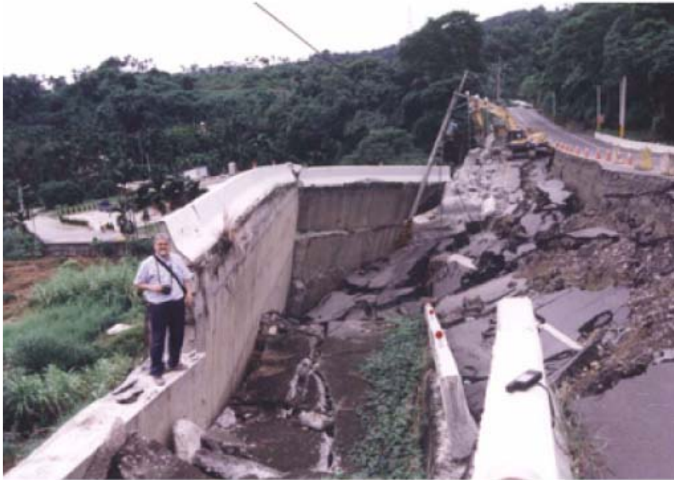
FIGURE 30.13 Gravity retaining wall pushed outward by landslide.
