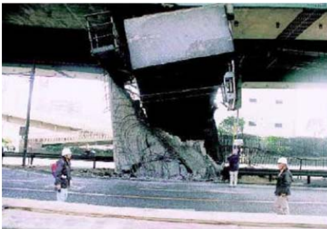
FIGURE 30.51 Shear failure of Pier 150 on Kobe Route 3.
