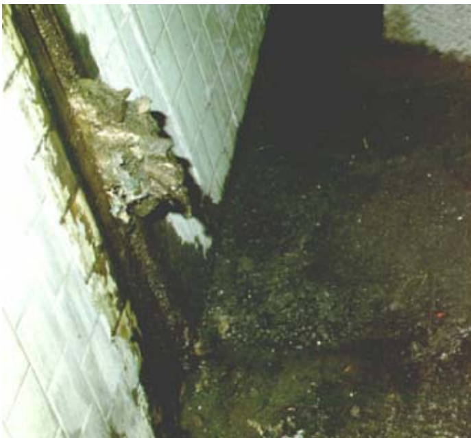
FIGURE 30.11 Liquefaction-induced damage to Webster Street Tube tunnel.
