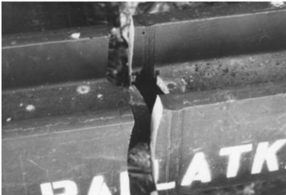
FIGURE 24.4: (a) View of jumbo section used as tension chord in a roof truss and (b) closeup view of fracture in web originating from weld access holes at welded splice.
