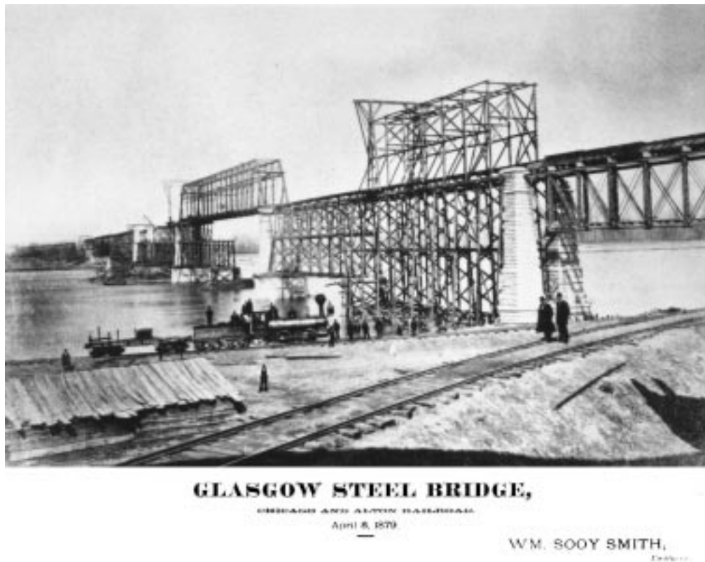
FIGURE 20.16: Glasgow (Missouri) railway truss bridge, 1879. Erection on full supporting falsework was commonplace in the 19th century. The world's first all-steel bridge, with five 315-ft (96-m) through-truss simple spans, crossing the Missouri River.
