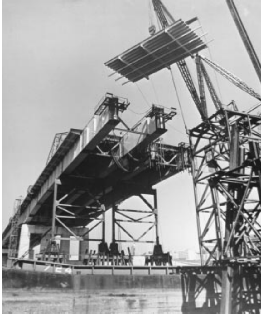
FIGURE 20.36: Erecting orthotropic-plate decking panel, Poplar Street Bridge, St. Louis, Mo., 1967. A five-span, 2165-ft (660-m) continuous box-girder bridge, main span 600 ft (183 m). Projecting box ribs are 5\frac{1}{2} \times 17 ft ( 1.7 \times 5.2 m) in cross-section, and decking section is 27 \times 50 ft ( 8.2 \times 15.2 m). Decking sections were field welded, while all other connections were field bolted. Box girders are cantilevered to falsework bents using overhead “positioning travelers” (triangular structure just visible above deck at left) for intermediate support. (Courtesy of Bethlehem Steel Corporation.)
