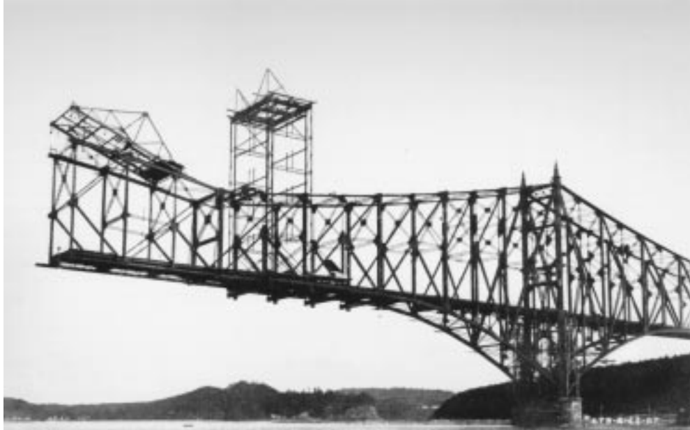
FIGURE 20.11: First Quebec railway cantilever bridge, 23 August 1907. Cantilever erection of south main span, 6 days before collapse. The tower traveler erected the anchor span (on falsework) and then the cantilever arm; then erected the top-chord traveler, which is shown erecting suspended span at end of cantilever arm. The main span of 1800 ft (549 m) was the world's longest of any type. The sidespan bottom chords second from pier (arrow) failed in compression because latticing connecting chord corner angles was deficient under secondary bending conditions.
