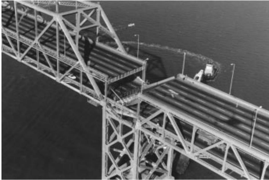
FIGURE 16.2: Aerial view of collapsed upper and lower decks of the San Francisco-Oakland Bay Bridge (I-80) following the 1989 Loma Prieta earthquake in California. (Photo by California Department of Transportation. With permission.)
