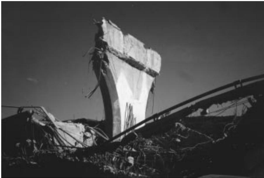
FIGURE 16.4: Collapsed SR-14/I-5 south connector overhead following the 1994 Northridge earthquake in California. (Photo by James MacIntyre. With permission.)
