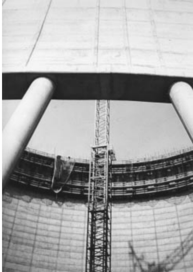
FIGURE 14.6: Climbing construction of the shell.
