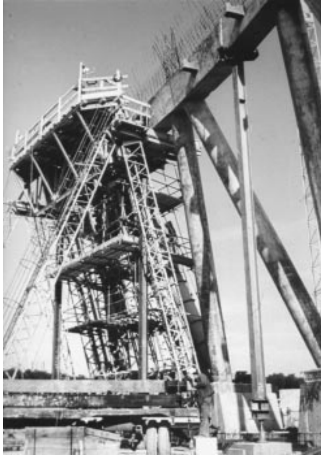
FIGURE 14.5: Fabrication of supporting columns.
