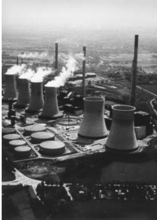
FIGURE 14.1: A group of hyperbolic cooling towers.
