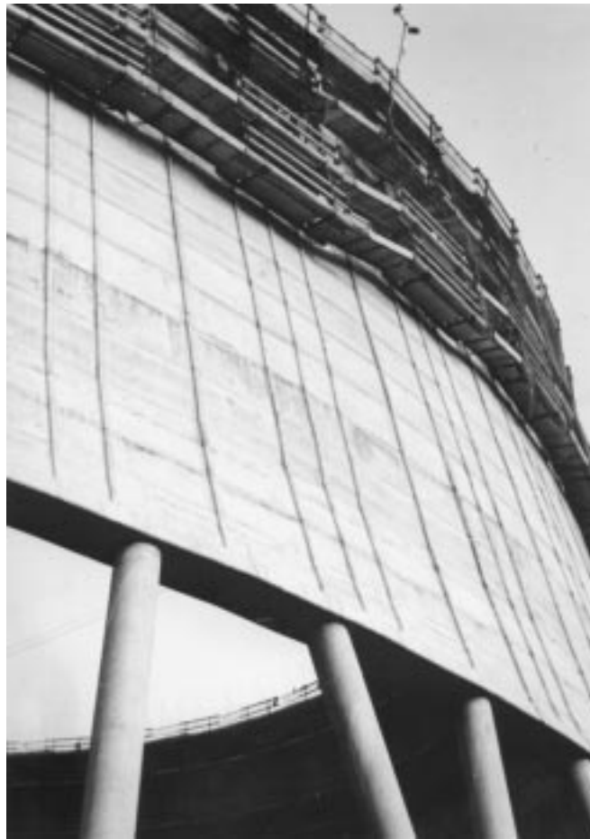
FIGURE 14.40: Column to lintel connection.
