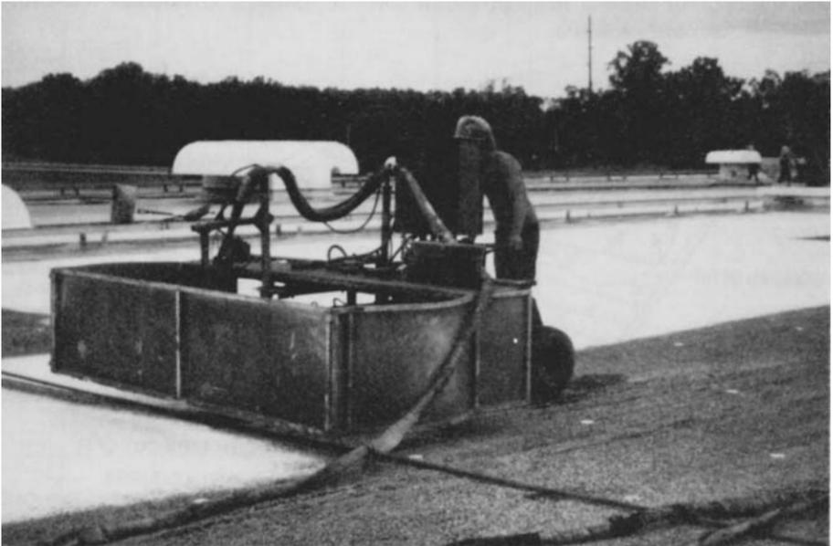
**FIGURE 12.6** Robotic sprayer applying polyurethane foam.
