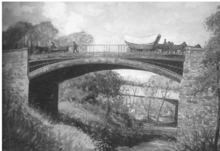
FIGURE 67.6 Dunlap's Creek Bridge, built in 1839, is the first iron bridge in the United States. It was built for the National Cumberland Road, at Brownsville, Pennsylvania, by Captain Richard Delafield of the Army Corps of Engineers. The bridge is still in service today. (Courtesy of Federal Highway Administration.)
