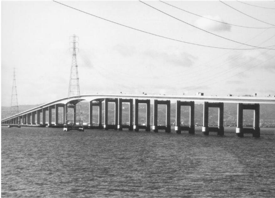
FIGURE 67.48 San Mateo–Hayward Bridge over the San Francisco Bay, not only has composite steel approach spans, but the main span has an orthotropic steel deck. Listed among distinctive bridges, it won an American Institute of Steel Construction prize in 1968. It was designed by the California Division of Bay Toll Crossings. (Courtesy of California Department of Transportation.)
