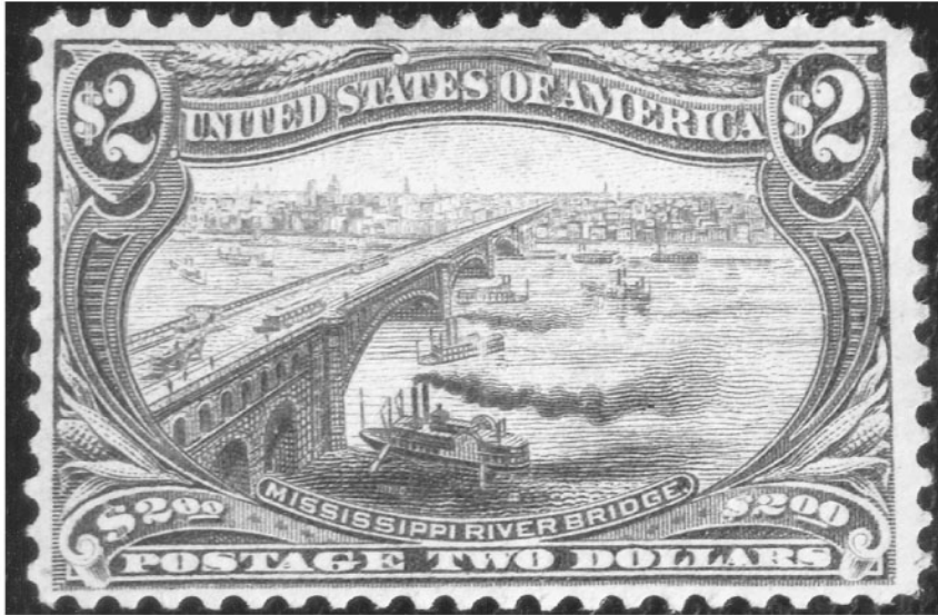
FIGURE 67.12 Eads' Bridge over the Mississippi River at Washington Street in Saint Louis shattered engineering precedents of the time. It was the first extensive use of steel for bridge construction. The three 175+ m arch spans are each four 464-mm steel truss-stiffened wrought iron tubes. The spandrels are extensive steel truss and lattice work. Built by James B. Eads in 1874. Eads' Bridge is pictured on the two dollar denomination United States postage stamp series commemorating the Trans-Mississippi Exposition of 1896. (Courtesy of U.S. Bureau of Engraving and Printing.)
