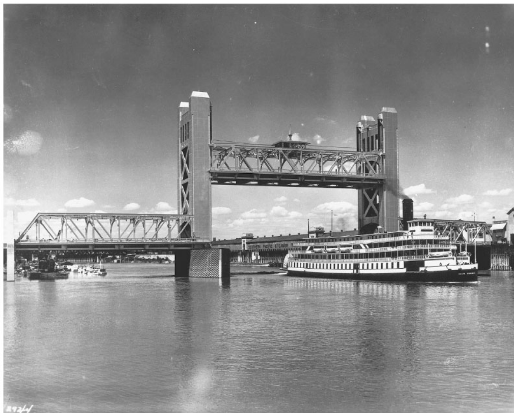
FIGURE 67.36 The Tower Bridge in Sacramento earned an AISC design award in 1936, the year in which it was built. This unique lift span is clad in steel plate to cover the moving parts. It was designed by Leonard Hollister of the California Division of Highways. (Courtesy of California Department of Transportation.)
