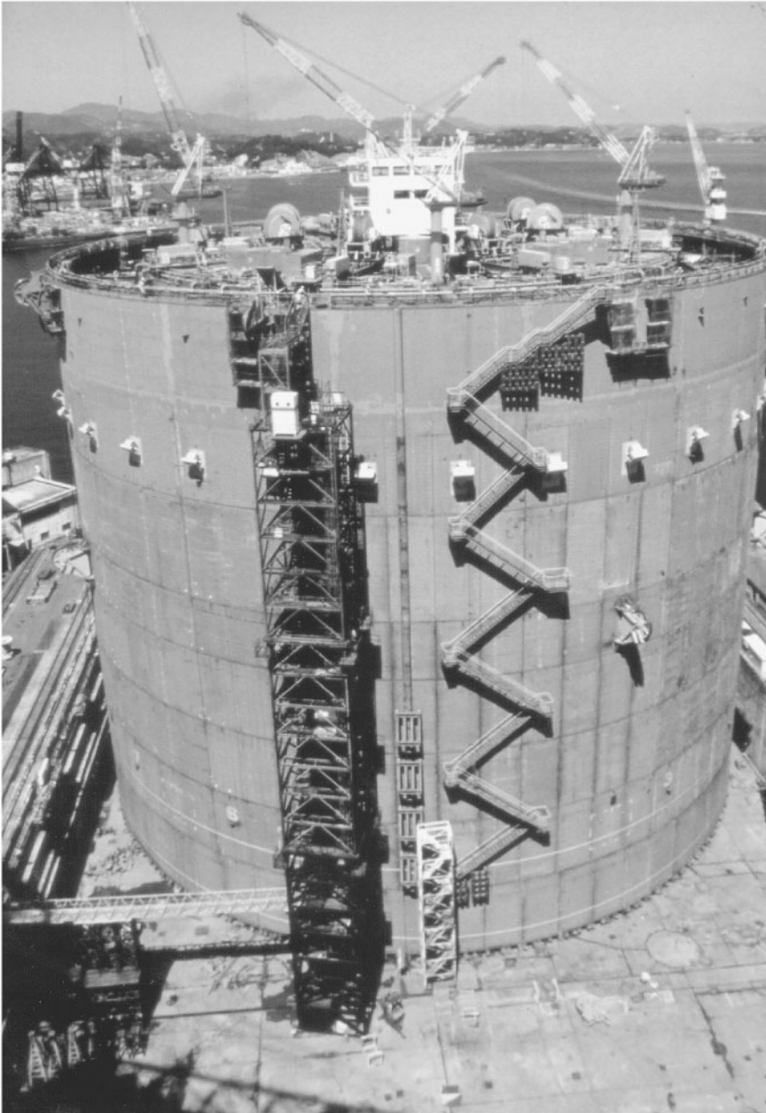
FIGURE 65.35 Steel caisson.
