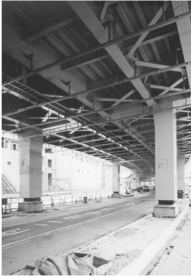
FIGURE 65.52 Rigid frame pier of Bente section. (Courtesy of Hanshin Expressway Public Corporation.)
