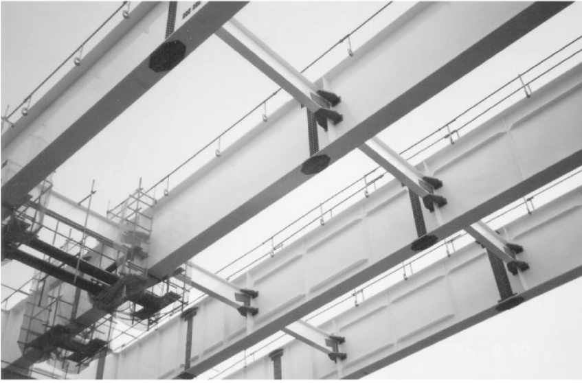
FIGURE 65.49 Plate I-girder with simple cross-beams.
