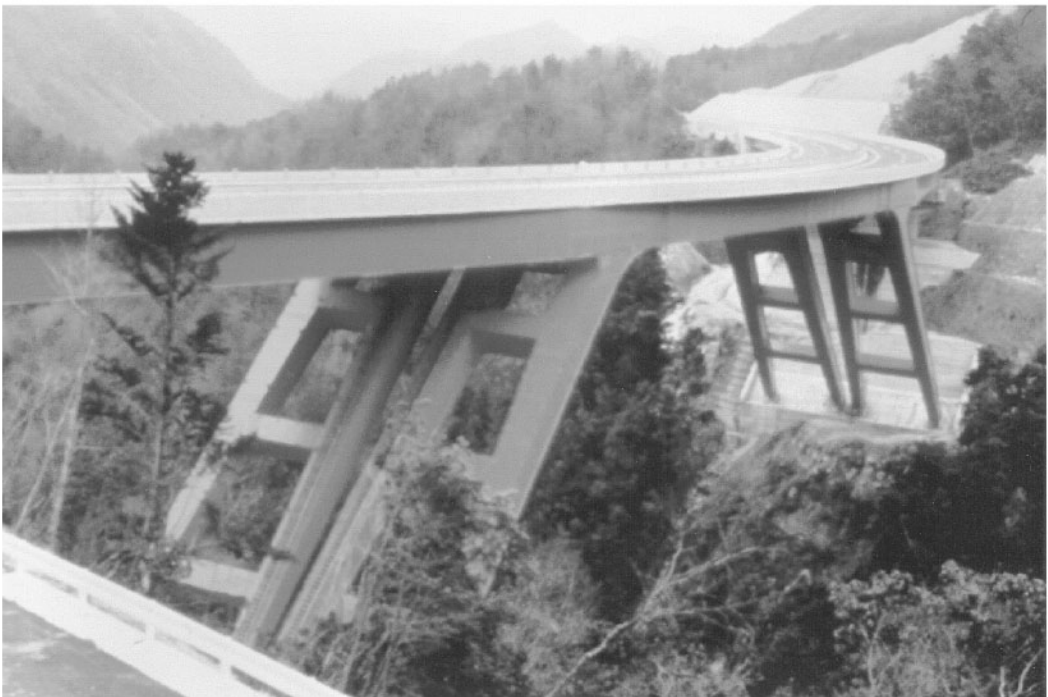
FIGURE 65.13 A typical \pi -shaped rigid frame bridge.
