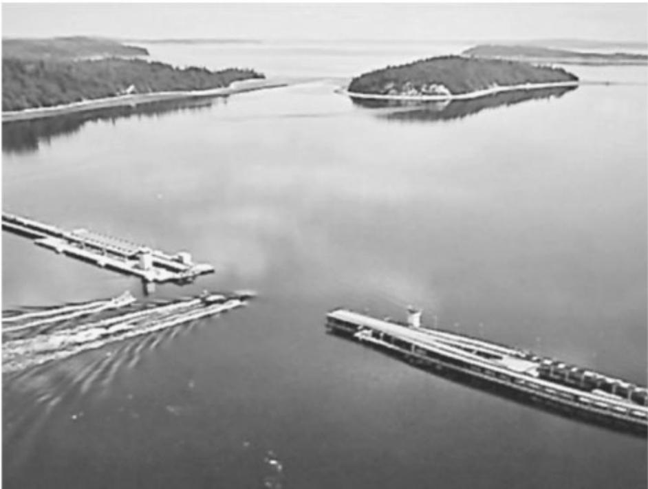
FIGURE 22.3 Movable spans for large vessels.
