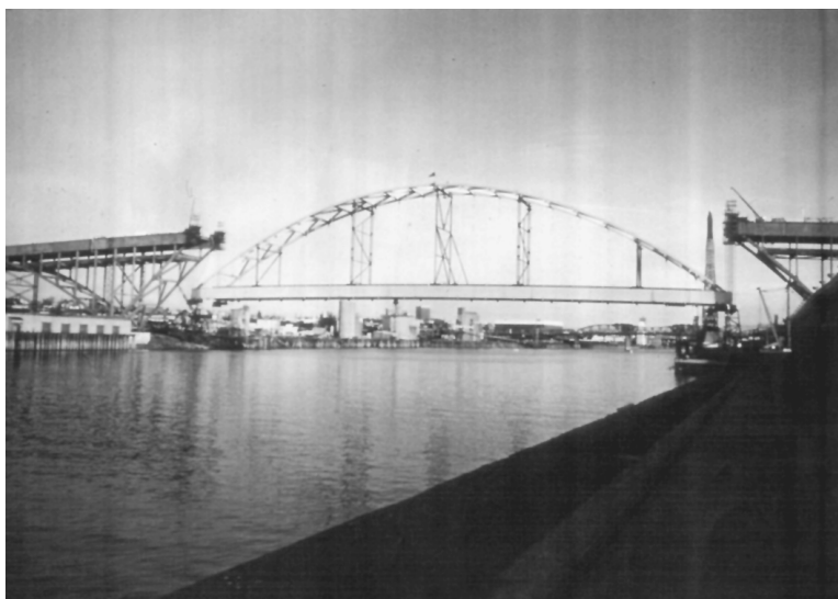
FIGURE 17.15 Fremont tied arch being lifted into place.
