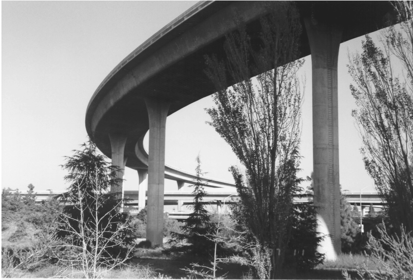
FIGURE 10.4 Prestressed box-girder bridge (I-280/110 Interchange, CA).
