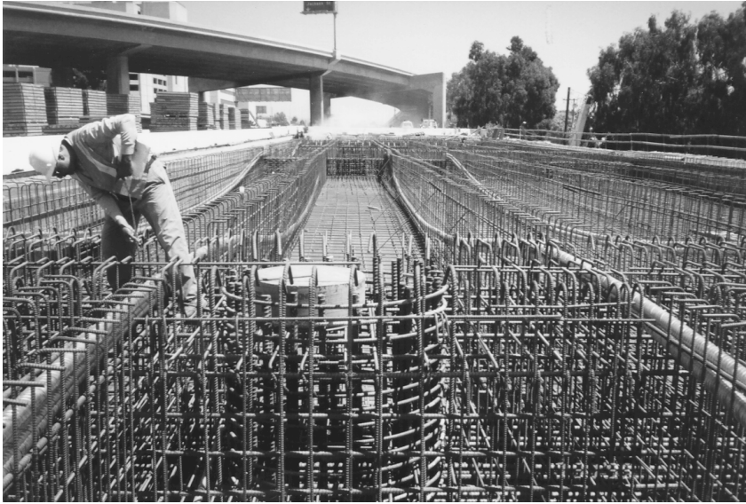
FIGURE 10.2 A post-tensioned box-girder bridge under construction.
