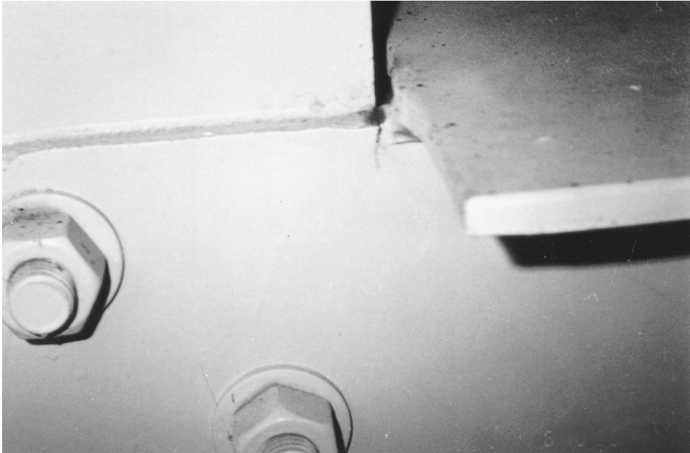
FIGURE 53.8 Close-up view of a crack originating at the termination of a flange on a floor beam with a “simple” connection to an attachment plate in the Dresbach Bridge in Minnesota. The crack is an indication of an end moment in the simple connection that is not predicted in design.
